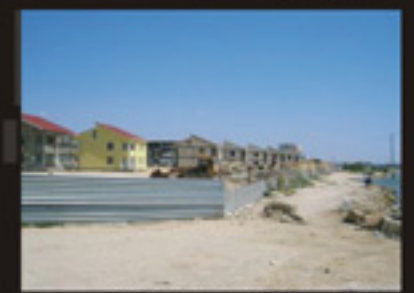
Settlement of individual homes (1st microdistrict)
