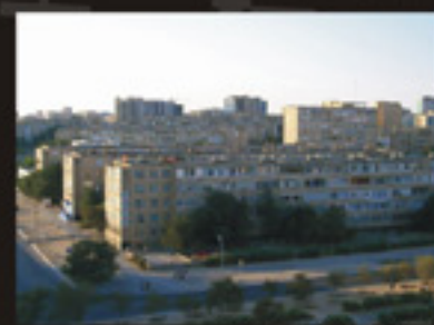
Row structures in the 4th microdistrict (2004)
