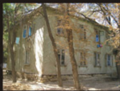
Wooden residential building in the 3rd microdistrict (2004)
