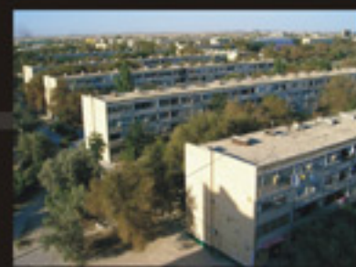
Row structures in the 1st microdistrict (2004)
