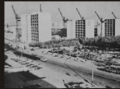
Erection of high-risers in the 1st microdistrict (around 1970)
