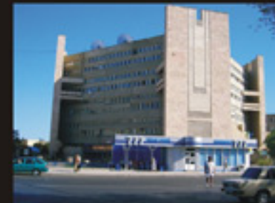
Telecommunications building (6th microdistrict)
