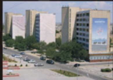
Typical ensemble of high-rise buildings with arcades (8th microdistrict)
